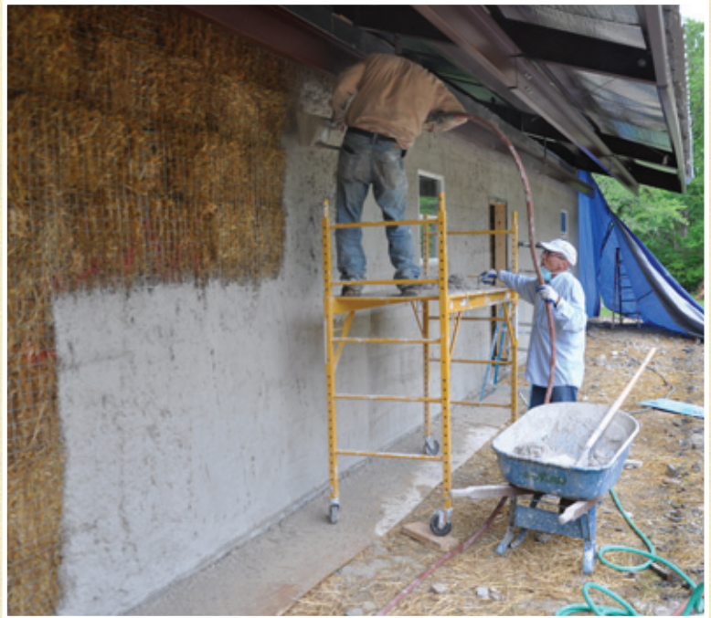
▲ Steve Wilson and David Gill applying the first coat of lime plaster to the exterior of Solar School's future home.
