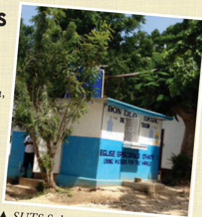
▲ SUTS Solar Panels power a school and clean water system in Trouin, Haiti.
